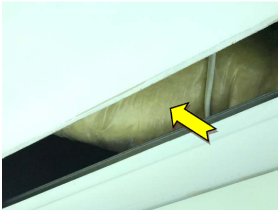
Photo 3. Interior, ground level, throughout above suspended ceiling – suspected SMF sarking insulation.
